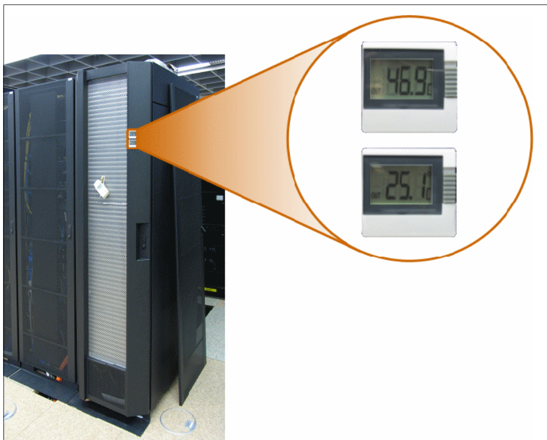
Figure 6 Rear door heat exchanger in action
