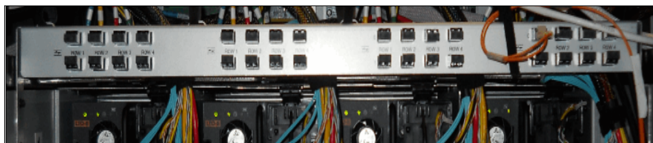
Figure 1-49 Fiber patch panel
